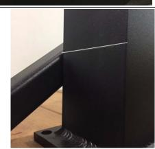
5. If the criteria are met in both steps 3 & 4, secure posts in place with the appropriate fasteners. Refer to page 1 of the post installation instruction details that are included with each post, regarding the proper fastening and securing of posts to the decking.
