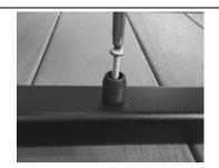
Cut 10" Support Block (F) to required length and press over the Support Block Connector installed in step 2. Support block is typically cut at 2" but can be cut longer based on your project needs.
