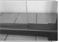
11. While holding the glass infill upright have an assistant place the 2nd piece of the rubber gasket material (K) on the top edge of the glass infill panel.
