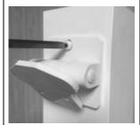
Note: Two screws are required to mount each bracket to properly secure in place. Depending on the post location, it may be necessary to temporarily remove the post or disassemble the hinge for adequate access to install the fasteners.
