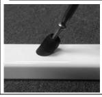
11. To assemble rail, begin with Top Rail (A) and insert balusters into each baluster hole. Use a rubber mallet to tap the balusters into place until fully seated into the Top Rail.
