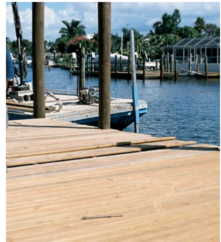
Elevated Service / Severe
