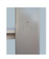
Next, hold the back plate on the centering mark, mark the two mounting holes. Also mark where the wire will feed through to get to the main feed line. TIP: depending on what style of post/ post sleeve you are using, the wire connections may be able to be made just under the post cap, or the pigtail wire may be able to slide between the post and the post sleeve to get to the joist and connect to the main line.
