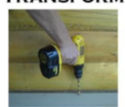
Drill a 3/8" hole through the deck surface and feed main line through to the under side of deck. Next, run the main wire to your first fixture. Secure the main wire using insulated staples or cable tacks. Tip: For faster installation pre-wire the main run before decking is installed!
