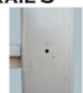
It is recommended that you predrill for the mounting screws to help not crack the surrounding material. Use a drill bit smaller than the screw to ensure the screw will hold. If passing the wire through and making connection under post cap or below the decking, use a 3/8" drill bit through the sleeve and into the space.
