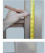
Determine where the fixture is to be installed and make a reference mark for centering the mounting and wire hole. Tip: measure from the top of the deck to the desired top of light height (usually around 34") and make a mark. Next, measure from left to right across the post and divide this # in half and mark. Center is where the two marks intersect.
