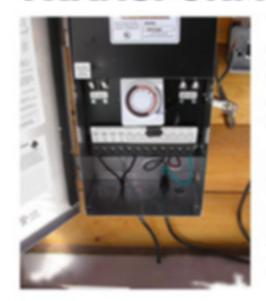
Using installation instructions provided with transformer, mount transformer to house and install main power feed line. This line should be a UV resistant, UL approved 12-2 low voltage cable with a 100' max run and no more than 250 watts. If run is more than 100' and over 250 watts, use 10-2 or 8-2 wire to carry the load. Be sure main line is long enough to reach the first lighting fixture.
