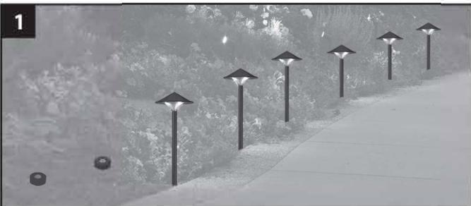
1 Locate placement of lights and lead wiring. If you choose to bury wire, under concrete or other permanent structures, plan accordingly.
