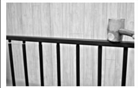
5. Locate bottom brackets in the Adjustable Gate Kit and slide each one onto the ends of the bottom rail with the counter bore holes up and facing toward the balusters.
