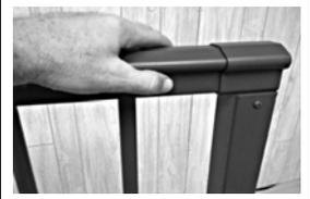
7. With the gate assembly hanging between the posts, place a mark on each of the posts at the point where the lowest part of the bottom bracket ends. Now remove the posts from the gate assembly and cut at the marked locations.
