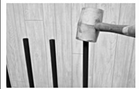
4. Attach balusters to bottom rail starting at one end and working to the opposite end. Stand unit upside down and firmly tap the bottom rail with a rubber mallet to secure the balusters in place.
