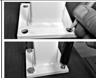
7. Remove the string line attached to saddle brackets. Reinstall the post base trim by sliding the trim over the top of the installed post down to the bottom of the post so that it covers the mounting flange.
