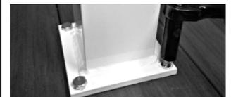
4. Install the post base trim by sliding the trim over the top of the installed post down to the bottom of the post so that it covers the mounting flange. Complete each rail section by installing the brackets and assembled rail per the instructions included with the rail kit.
