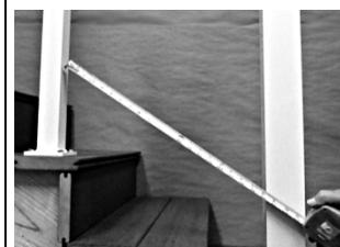
9. Place the bottom rail which has been cut to length, parallel to the top rail aligning the baluster connectors, transfer the cut length to the top rail. Cut the ends of the top rail that will mount into the Over-the-Post Top Rail Bracket at the marked position. Cut an additional 5/8" of material from the end of the top rail (as shown in the photo) that will mount into the Top Rail Saddle Brackets on the upper and lower post. All cuts should be made at the same 34° angle.
