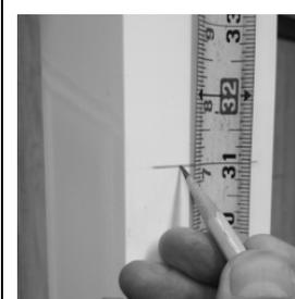
6. Align screw holes in the upper and lower saddle brackets (C&D) on the marked lines. Make sure the brackets are centered on the posts. Mark the screw hole locations with a pencil.
