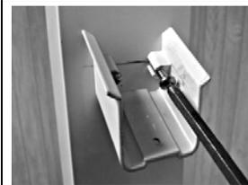
8. Install support block connectors (I) using 1-1/2" self-drilling screw (J) to the underside of bottom rail (B). The support block (H) will be installed in step 13.
