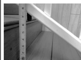
14. Slide and hold the upper bottom bracket (F) firmly against the top post. Secure the bracket with 1-1/2" self-drilling screws (J). Repeat the process securing lower bottom bracket (G) to the bottom post using 1-1/2" self-drilling screws (J).
