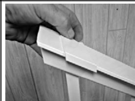
12. Slide bottom brackets (F&G) with the counter bore holes facing down and toward the balusters, over each end of the bottom rail (B). A small piece of tape may be required to hold lower bottom brackets in place. Next, set the rail assembly into the saddle brackets (C&D) letting the bottom rail hang freely between the posts.
