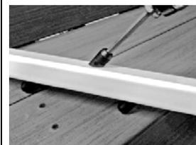
9. To assemble rail, begin with top rail (A) and insert balusters over pre-installed connectors. Use a rubber mallet to tap the balusters into place.
