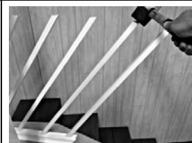
10. Attach balusters to bottom rail (B) beginning at one end and working to the opposite end. Stand the assembly upside down on the surface of the box and tap the bottom rail with a rubber mallet to secure the balusters in place. Stand assembly upright.
