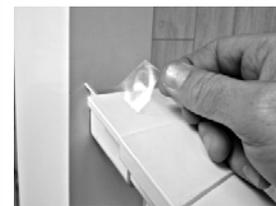
16. Screw 1-1/2" self-drilling screws (J) into the top rail (A) from the underside of saddle brackets (C&D) through the provided locating hole.
