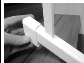
13. At the point(s) where you installed support block connectors (step 8), carefully measure the distance from the underside of the bottom rail (B) to the floor. Cut support block material (H) to fit. Slip support blocks over support block connectors (I). Slide the rail back into place and make certain the rail is plumb.
