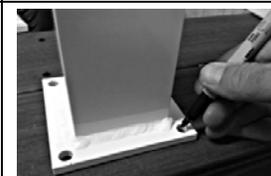
3. Remount the post assembly. Insert the appropriate fasteners then secure the base to the deck structure. Make certain the posts are plumb. If the post requires adjustment, add stainless steel washers under the base plate. Do not install the base post trim and post capitals until step 4 of the rail installation.
