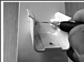
7. Attach saddle brackets (C&D) with 1-1/2" self-drilling screws (J) at the marked screw locations in step 6. Pre-drilling is recommended.
