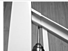
17. If a deck board is to be installed on top of the rail, carefully measure and cut the material to the length required. Place the deck board on top of the rail and secure from the underside of the rail as shown, with the appropriate fasteners under the flange of both sides of the rail.
