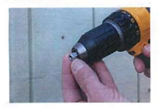
1) Lock the *Installation Tool* into the chuck of a ½" electric drill (or use 3/8"socket wrench).
