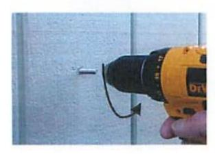
4) Reverse the spin direction of the electric drill to free the Hanger Bolt from the *Installation Tool*.
