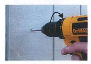
Using a low speed, drive the Hanger Bolt into the pilot hole (or Masonry anchor) to the recommended depth.
