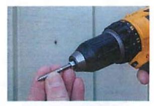
Spin the machine thread end of the Hanger Bolt all the way into the *Installation Tool*.
