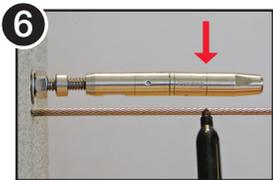
6 Stretch cable tight across fitting and mark at Cut Gauge Line. Cut cable at mark.
