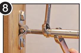
8 Tighten the lock-nut against the swivel portion to prevent the fitting from loosening.
