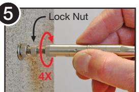
5 Spin the turnbuckle lock-nut onto the exposed threads. Then attach Quick-Connect® and rotate the body 4 full turns.
