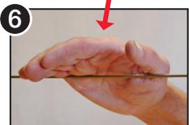
6 Hand tighten the turnbuckle as far as possible, then swiftly hit the cable line with your palm several times to ensure that jaws are securely seated.
