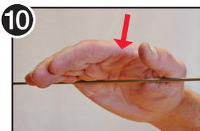
10 Hand tighten the turnbuckle as far as possible, then swiftly hit the cable line with your palm several times to ensure that jaws are securely seated.
