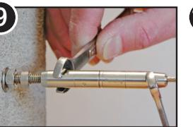
9 Use wrenches to tighten the Turnbuckle to desired final tension.
