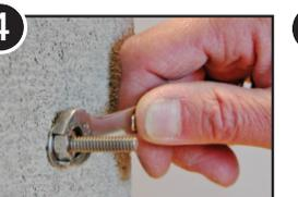
4 Use 7/16" wrench to tighten anchor nut until anchor is properly seated and locked.
