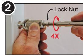
2 Spin the turnbuckle lock-nut onto the threads. Then attach the Quick-Connect® and rotate the body 4 full turns.
