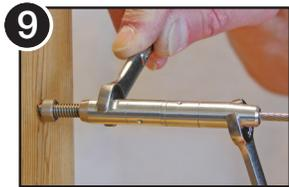
9 Use wrenches to tighten the Quick-Connect® to desired final tension.
