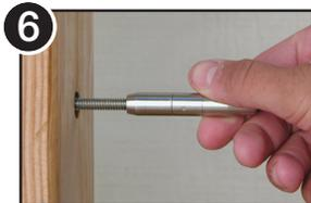
Spin Quick-Connect® onto Hanger Bolt until it bottoms out.
