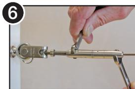
6 Use wrenches to tighten the Quick-Connect® to desired final tension.
