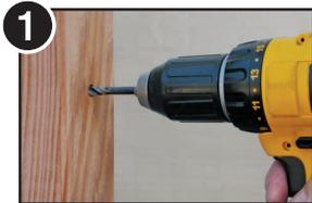
Drill 7/64" pilot hole (7/32" hole for 3/16" fitting). Harder woods may need larger hole.
