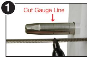
Stretch the cable tight. Mark with felt pen at Cut Gauge Line.
