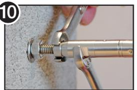
10 Tighten the lock-nut against the swivel component to prevent the fitting from loosening.
