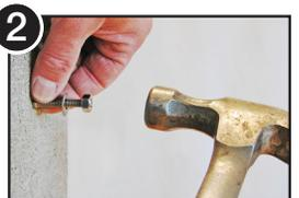
2 Carefully tap the Expansion Anchor (with washer and anchor nut).
