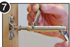
7 Use wrenches to tighten the Quick-Connect® to desired final tension.
