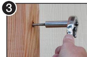
Drive Hanger Bolt into post using socket or electric drill.
