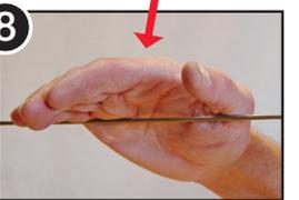
8 Hand tighten the turnbuckle as far as possible, then swiftly hit the cable line with your palm several times to ensure that jaws are securely seated.
