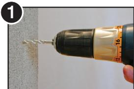
1 Drill 1/4" hole with masonry bit to 1-1/4" (minimum) depth. Blow debris out of hole.
