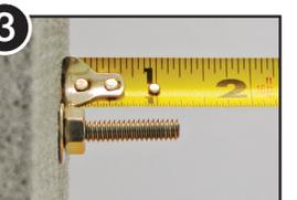
3 Tap until approximately 1-1/4" of the threaded shaft protrudes from the wall.
