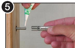
5 Apply a drop of high strength thread locking compound to machine threads of the hanger bolt.
