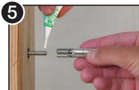
Apply a drop of high strength thread locking compound to threads.
